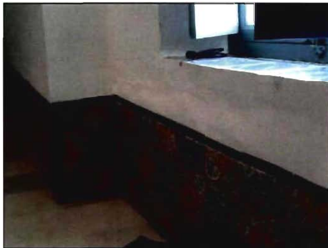
Figure 35 : Couloir, Dar Abassi.
