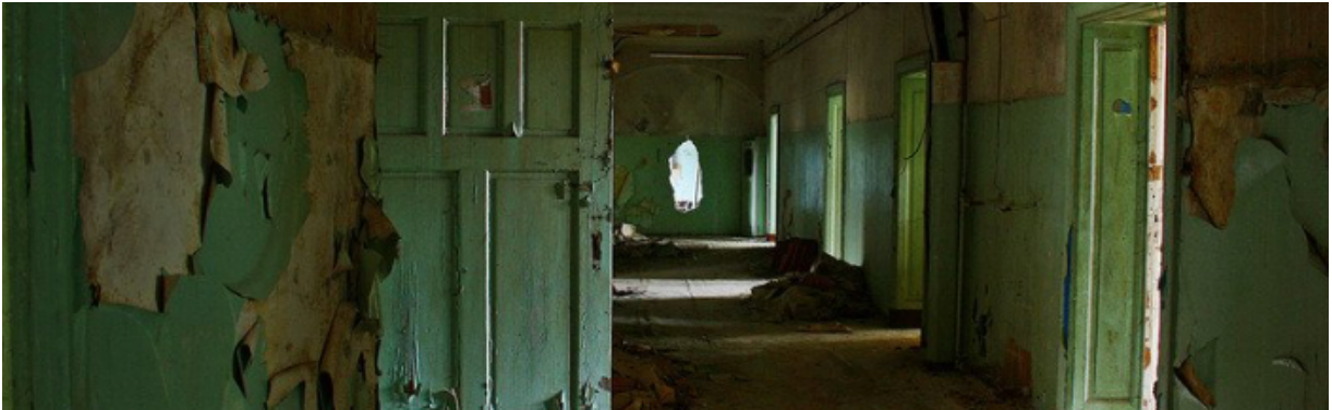
Figure 40 SIFotografie, Abandoned residential building, 25 janvier 2015.
