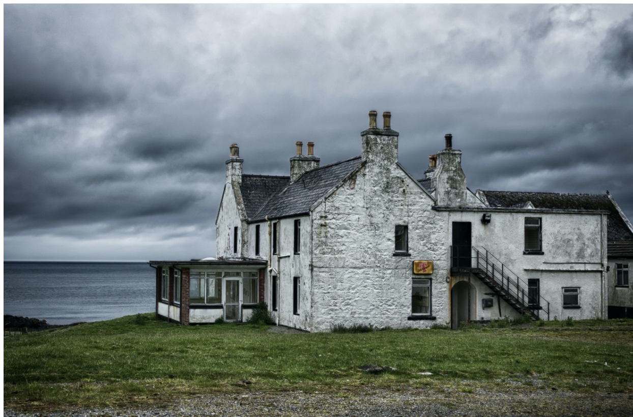
Figure 46 Tama66, Abandoned house by the coast, 10 juin 2017.
