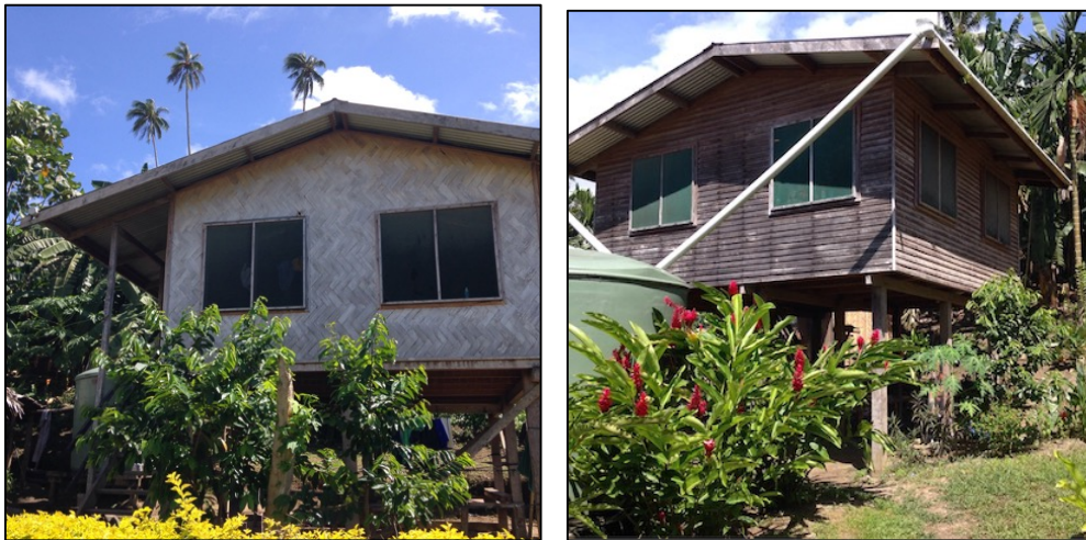
Figure 10. Finished houses on the relocation site in Tinputz
