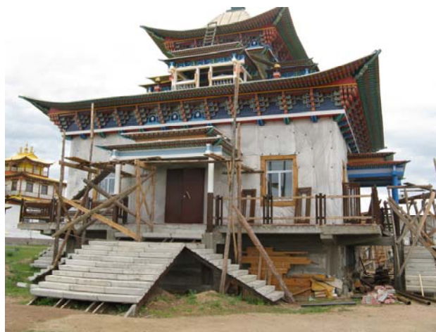
Figure 4: Buddhist temple in construction (I. Kaneva, 2009)
