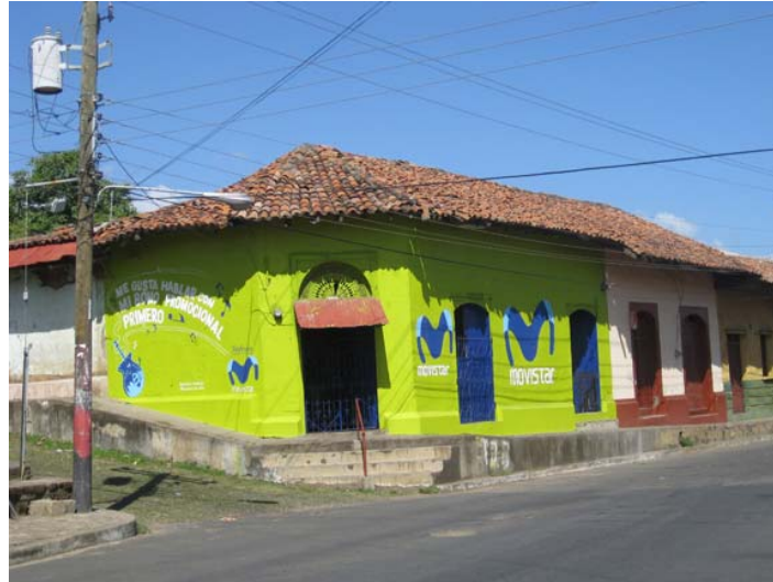
Figure 3: Electrical accessories store in the historic center of León (M. St-Denis, 2009)
