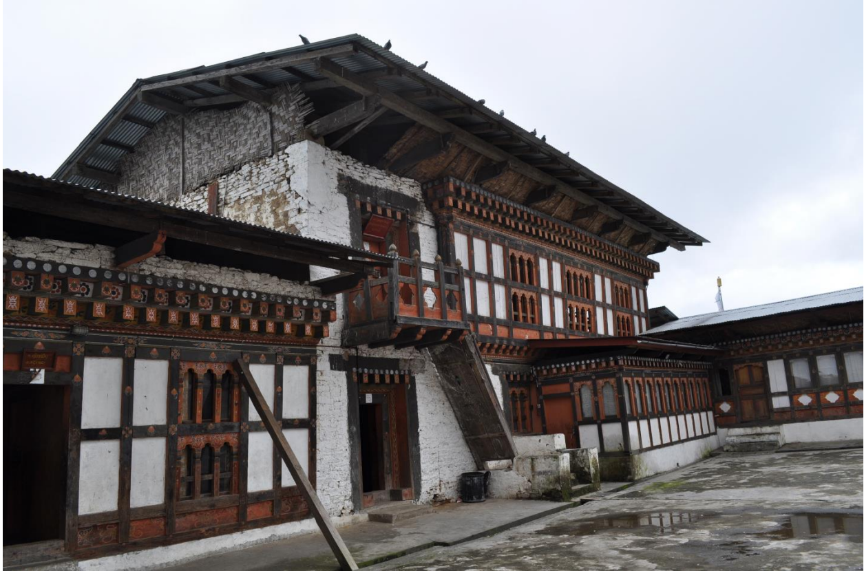
Drametse Lhakang Shakor, Bhutan, post-earthquake (Image: Stephen Kelley/World Monuments Fund)
