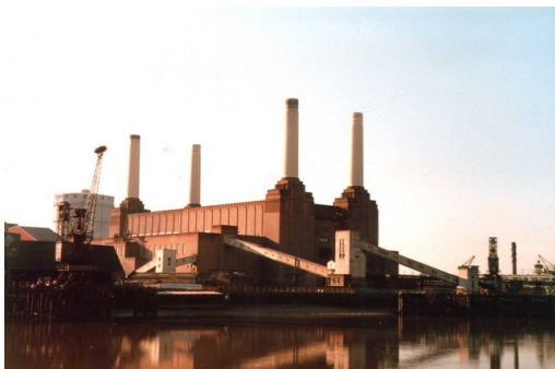
Fig.30. Evans, K. Battersea Power Station . Nov. 1986. Wikimedia Commons . 12 dec. 2016. < https://en.wikipedia.org/wiki/File:Battersea_Power_Station_-_geograph.org.uk_-_794104.jpg >
