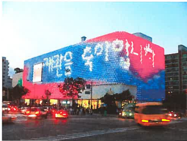
Figure 15: Arup Lighting and UN Studio's LED screen for the Galleria West fashion mall in Seoul, South Korea
