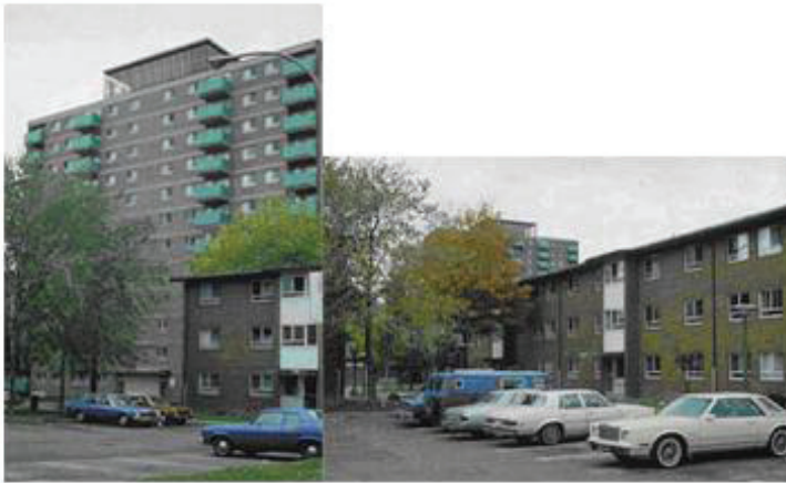
Rother, Bland, Trudeau, urban planning consultants, Greenspoon, Freedlander, Dunne, with Jacques Morin, architects, Ian MacLennan, consultants, Les Habitations Jeanne-Mance, 1960.
