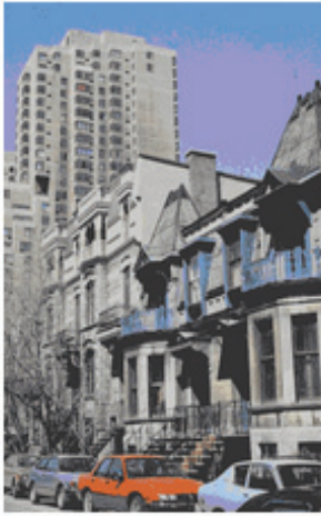
Milton-Parc Coop, Montréal. Cooperative and neighbourhood conservation group formed as a reaction to a high-rise housing development.
