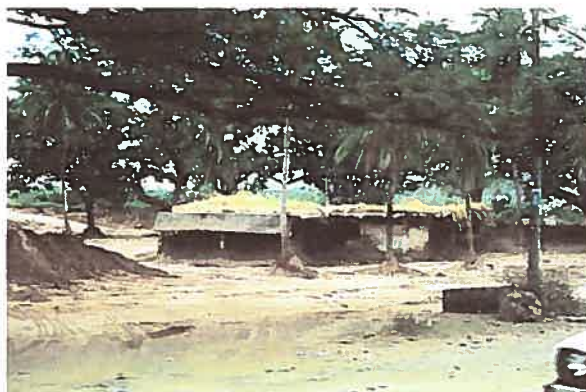
Fig. 3.12 Gas station in Choluteca just after Hurricane Mitch. Source: http://www.agenvsafety.tamu.edu
