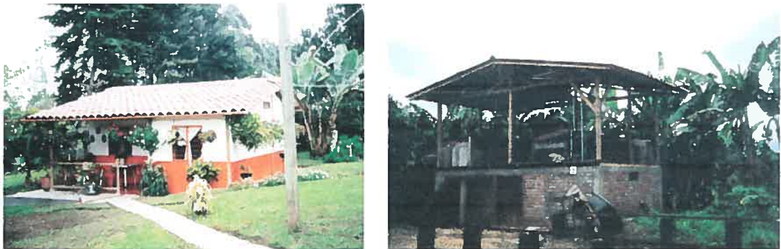
Fig. 3.9 Self-help made constructions. Left: house built using pre-fabricated components; the design corresponds to the prototypes proposed by the CGOs. The layout, scale, distribution and multiple details correspond to traditional vernacular housing in the region. Right: Customised structure for processing coffee beans (called "beneficiadero").
