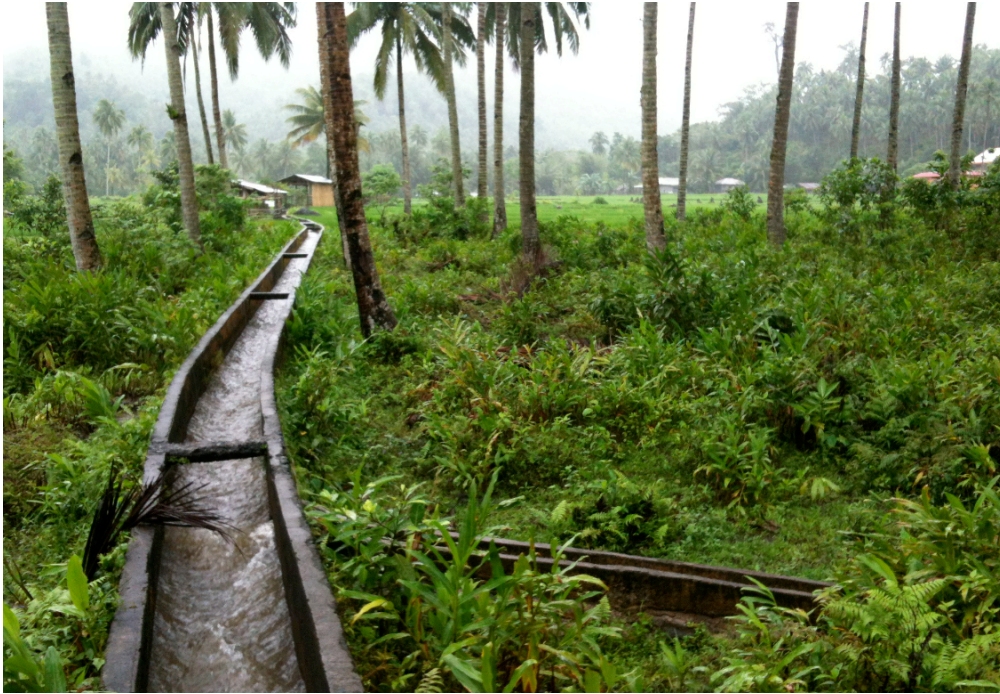
Picture V.7. Irrigation in Saint Bernard (Source: Veuthey 2013)
