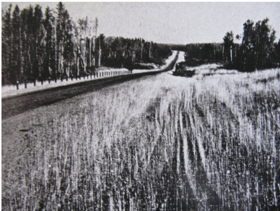
Figure 64 : « Typical growth after seeding operation, Highway 11 ». Source : Ontario, Annual Report of the Department of Highways of Ontario for the fiscal year ending March 31 st 1954 , Toronto, 1954, p. 21.
