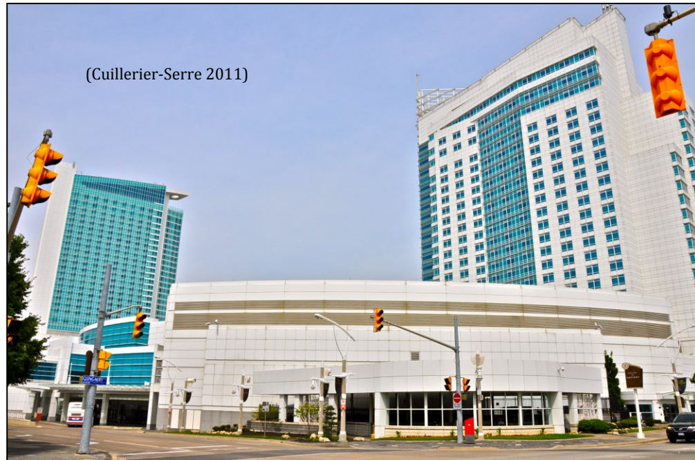
FIGURE 1,2 : CEASAR'S CASINO, CENTRE-VILLE DE WINDSOR
