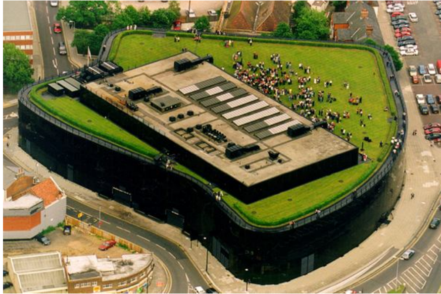
Figure 3.14 Willis Building in Ipswich (UK) (Copyright © 1975, Foster and Partners)
