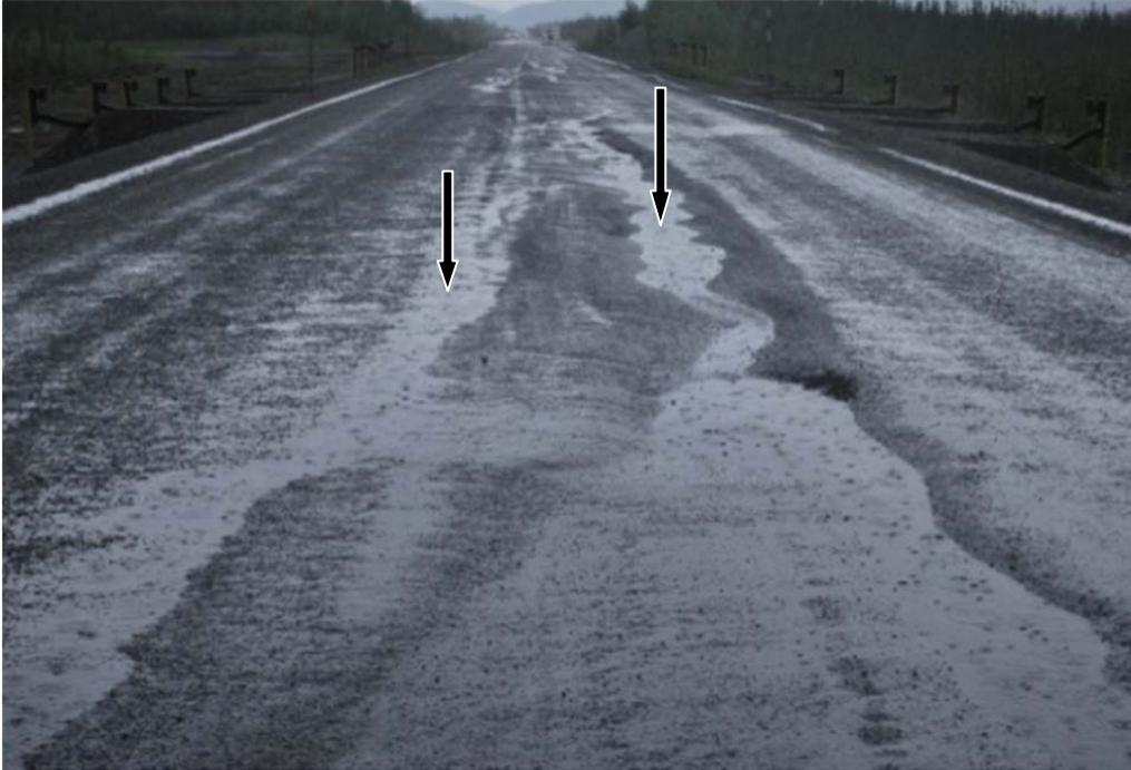
**Figure 9. Depressions in the road (black arrows) at the study site are outlined by water accumulation during a rain event. The road is 15 m wide.**
