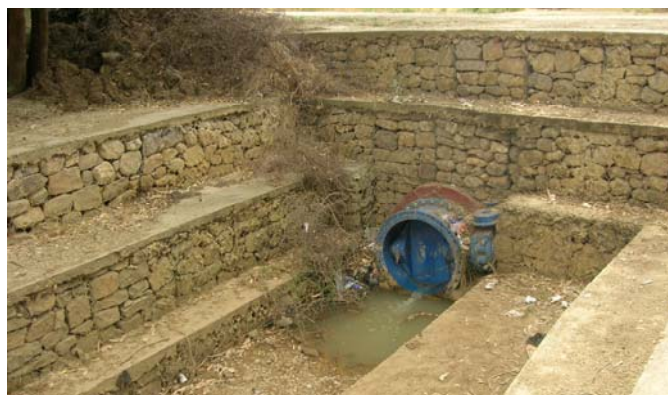
Figure 3.9 Clapet anti retour. (Photo : Bouraoui, 2009-06-02)
