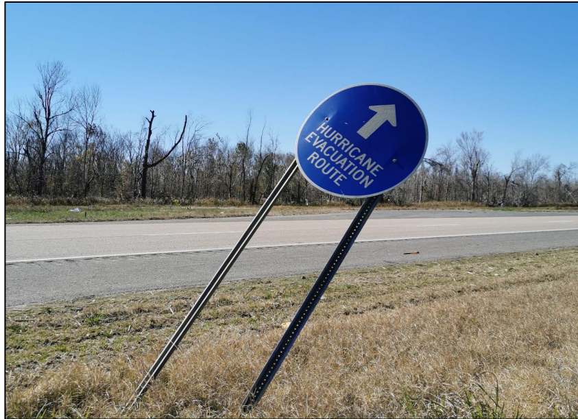
Photo 10. - A bent hurricane evacuation route sign after the passage of Hurricane Ida
