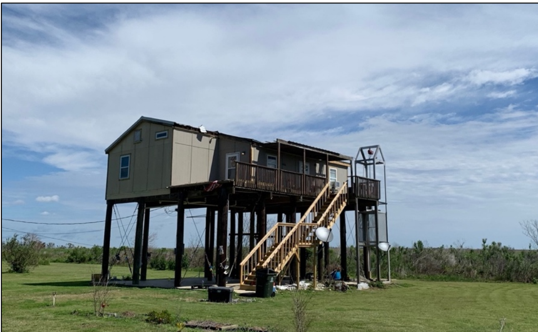
Photo 18. - Elevated home with a lift on Isle de Jean Charles, Terrebonne Parish
