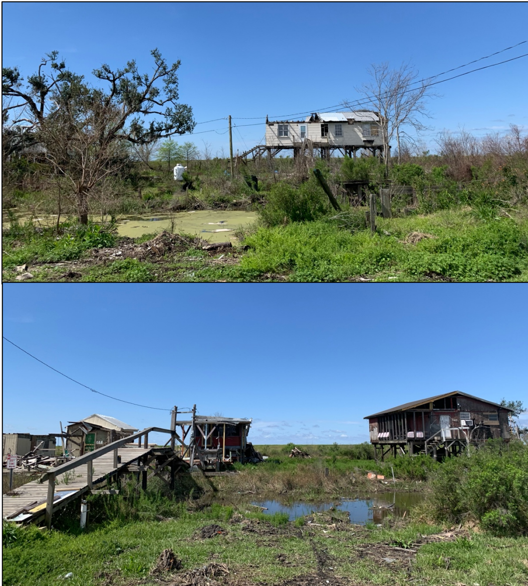
Photo 25. - Houses damaged by Hurricane Ida on Isle de Jean Charles
