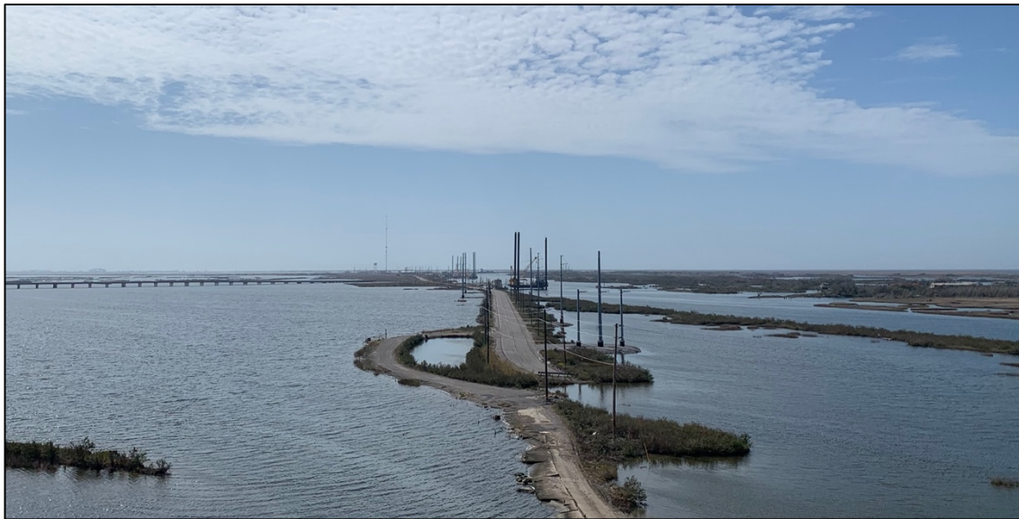
Photo 6. - View of the submerged road below the LA-1 highway, towards Port Fourchon
