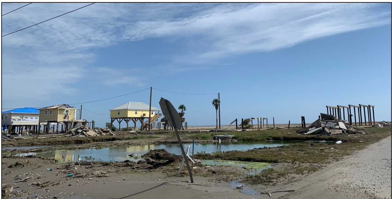
Photo 15. - Damage from Hurricane Ida in Grand Isle
