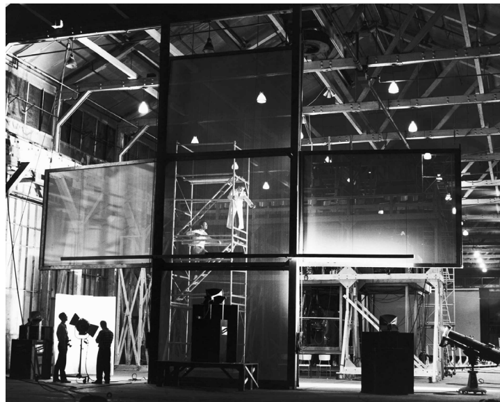
Photograph of the construction of the multi-screen in the third room of the Labyrinth pavilion. See database entry.
