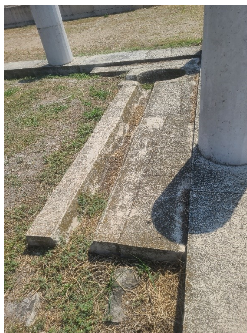
Fig. 30- Water conduits and basins, Agora, Pella. (Personal Archive)
