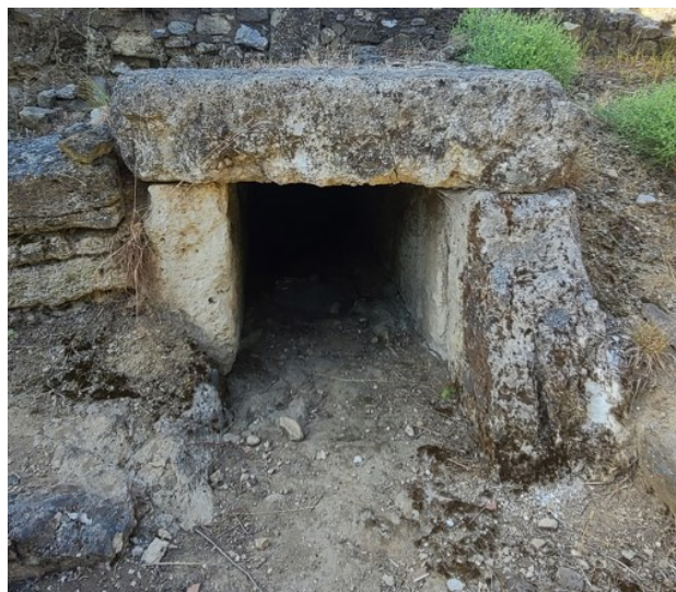
Fig. 29- The interior of the primary sewer system, Gymnasium , Amphipolis. (Personal Archive)
