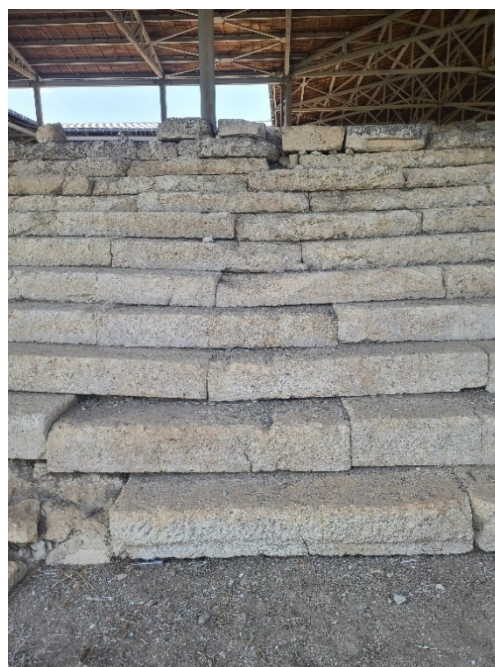
Fig. 19- Eastern Staircase with marks from consistent water drainage, Gymnasium , Amphipolis (Personal Archive)
