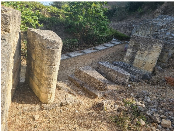
Fig. 54- Water conduits, Northern fortifications, Amphipolis. (Personal Archive)
