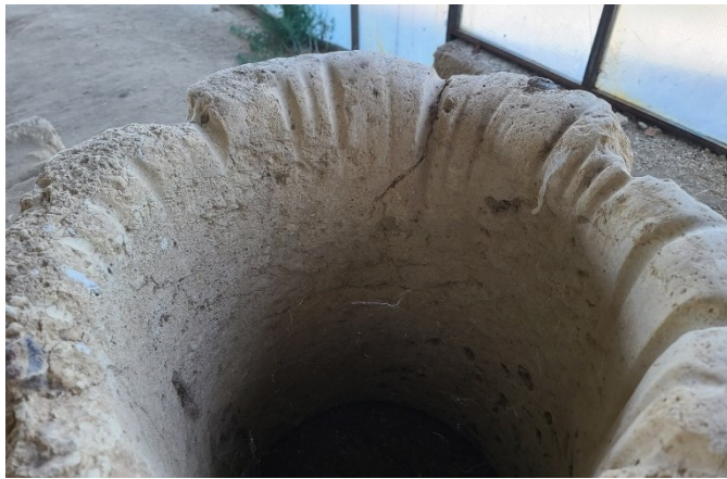
Fig. 1-Terracotta cylindrical lining for well, Dion (Personal Archive)
