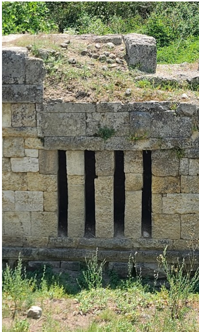
Fig. 56- Water evacuated with a conduit allocating water from specific areas. A- Exterior face of water conduit. B- Interior channel leading to water conduit. Northern fortifications, Amphipolis. (Personal Archive)
