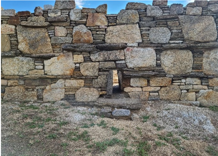
Fig. 52- Vertical water evacuates in the fortification, Acropolis, Stagira. (Personal Archive)
