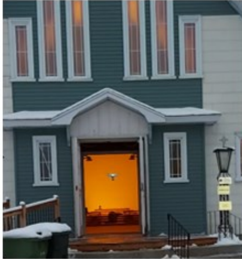
Entering a building
