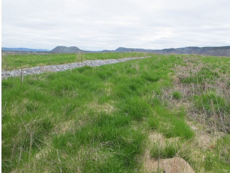
Figure 3. – The plateau of a waste rock pile seeded with grasses on a technosol made of a mixture of by-products at an asbestos mine in southern Quebec. Credits: N. Bélanger
