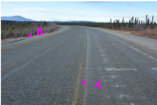
(c) Asphalt-paved surface of embankment center
