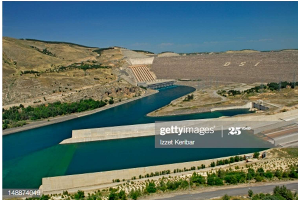
Figure 3. Atatürk Dam. – Photos, Sanliurfa, Turkey, Middle East (Photo: Izzet Keribar / The Image Bank Unreleased via Getty Images).
