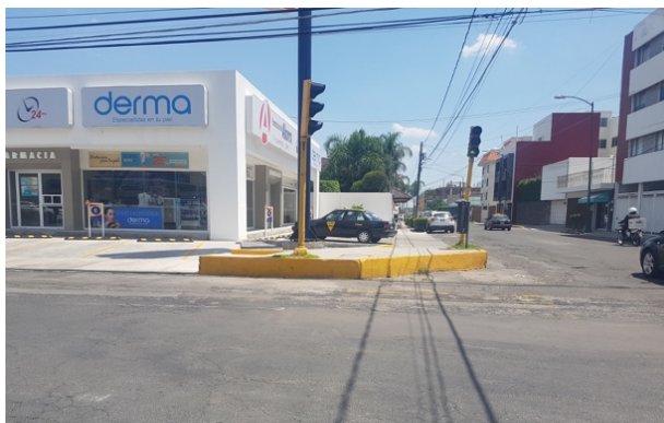
Figure 15: Cut corner and absence of pedestrian infrastructure
