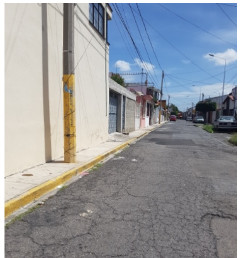
Figure 25: Narrow sidewalk obstructed by utilities pole
