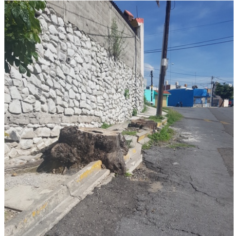
Figure 24: Sidewalk obstructed by pole and tree stumps
