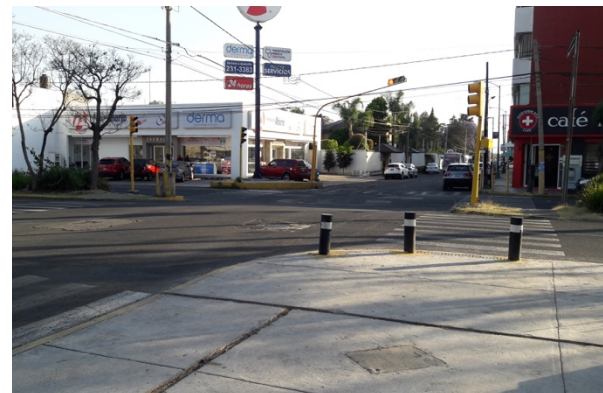
Figure 16: Intersection after improvements
