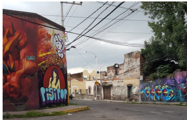
Figure 11: Degradation and vandalism in El Refugio
