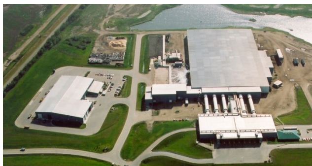
Figure 1.10. Edmonton composting facility (taken from an open access source). 7
