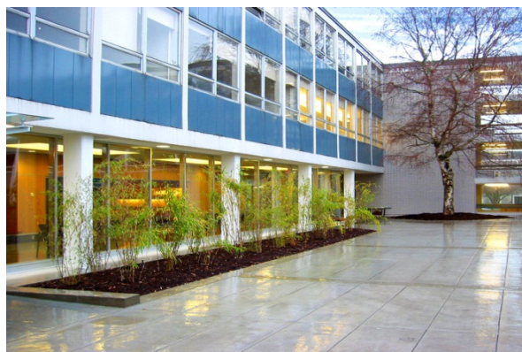
Figure 4- Buchanan Complex after Rehabilitation.
