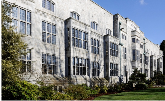
Figure 3- UBC Chemistry Building after Rehabilitation.
