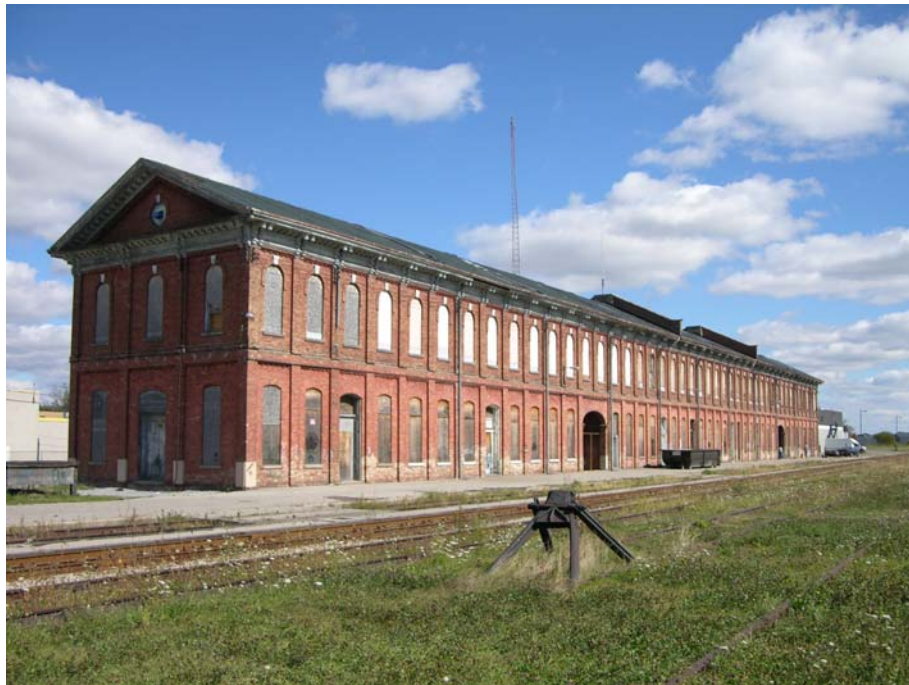
Figure 2- The Former Canadian Southern Railway Station Built in 1873 in St. Thomas, Ontario. Restoration of this federally-designated and now provincially protected historic site started in 2007 and continues to this day using labour intensive traditional technology and trades. (Photo Credit: Sean Fraser, 2004).
