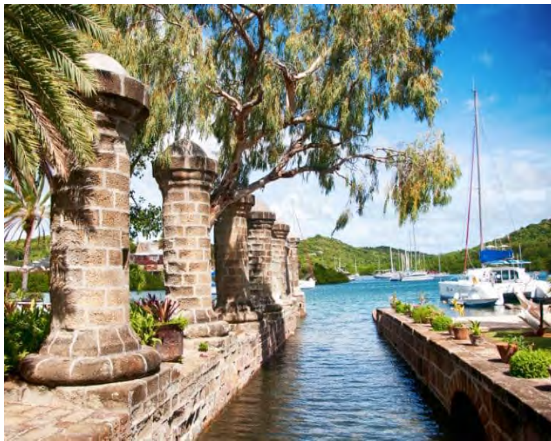
Existing Docking Facility
