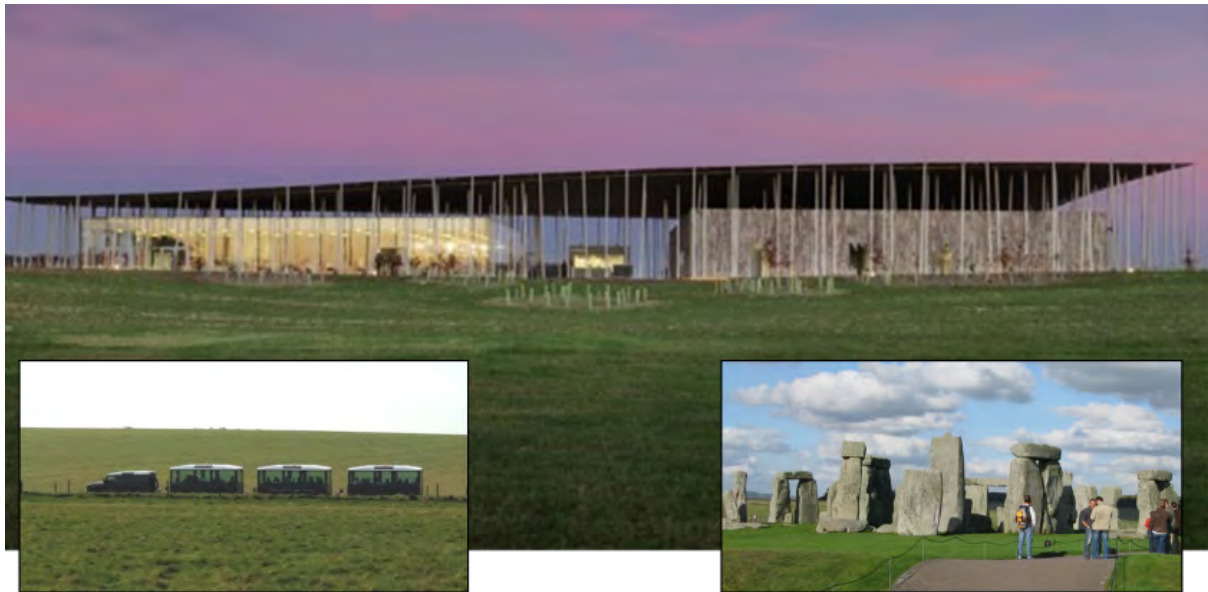
Stonehenge Visitor Centre – Architects: Denton Corker Marshall – with land train to the Neolithic stones
