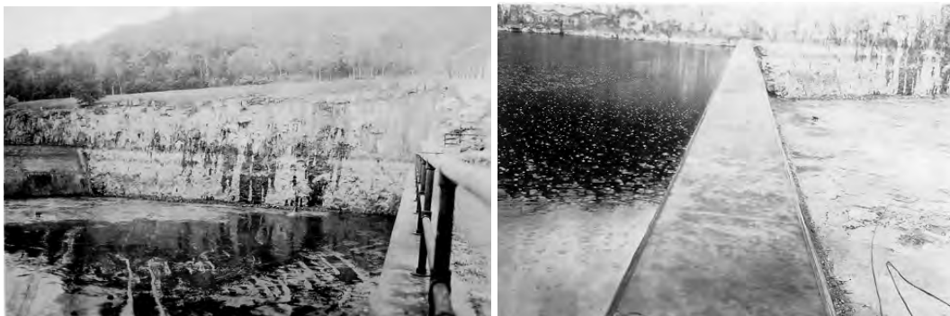
Figures 3.5-3.6 Outremont basin being cleaned ca. 1951
