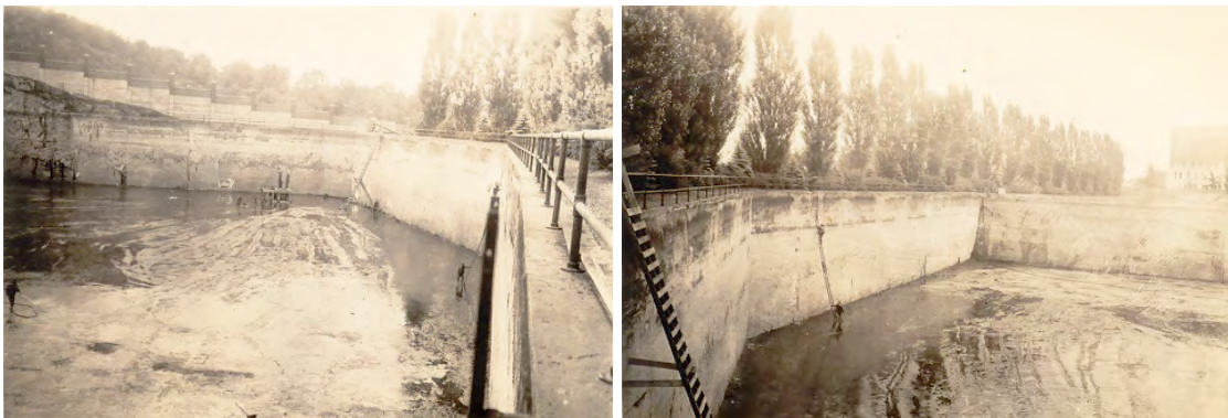
Figures 2.30-31 Outremont basin being cleaned, ca. 1951
