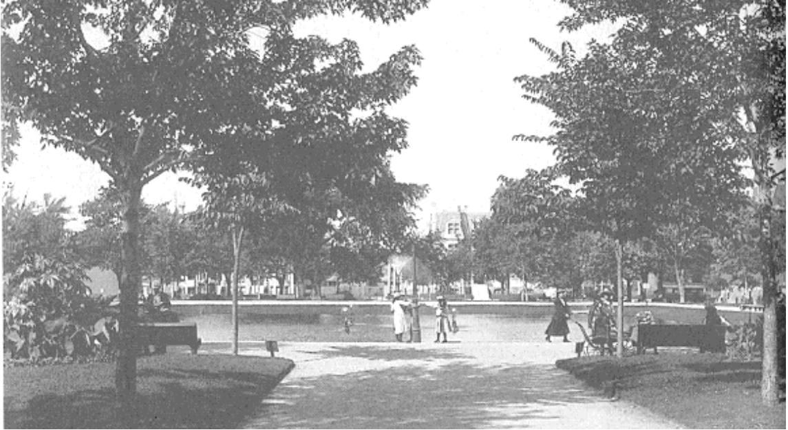
Figure 2.15 Saint-Louis Square with reservoir basin, ca. 1895
