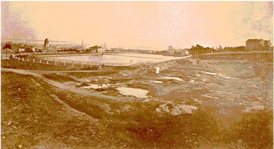
Figure 2.22 “McTavish Reservoir M.W.W.” ca.1873 Original elliptical form with quarry for extension to northwest (right in photograph)
