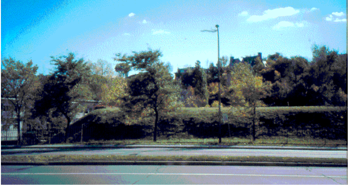
Figure 2.5 Côte-des-Neiges reservoir from Côte-des-Neiges Road, 2001
