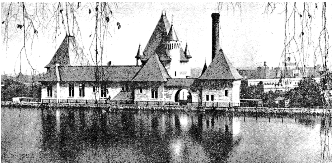
Figure 2.36 McTavish reservoir and pumping station, ca. 1937
