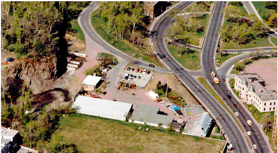
Figure 5.11 Aerial photograph of Côte-des-Neiges reservoir site, 1996
