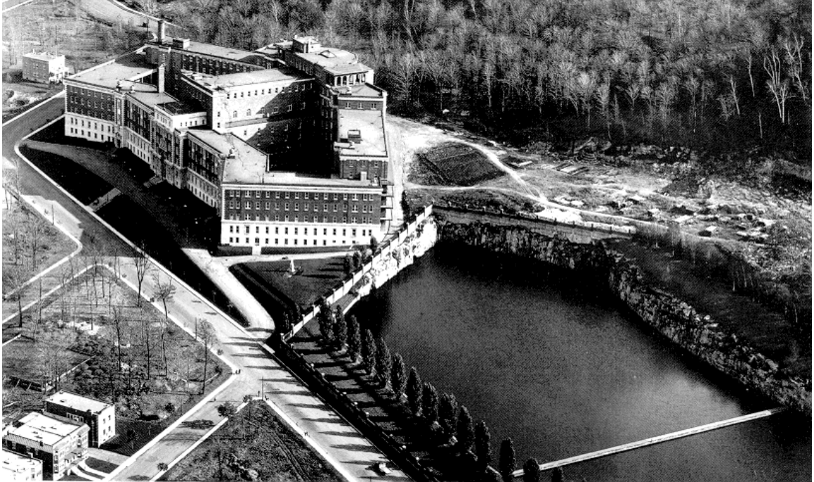
Figure 2.29 Outremont reservoir, ca 1930
