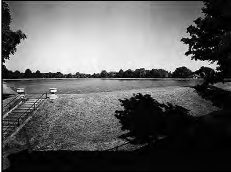
Figure A.24 Rosehill reservoir, 1955
