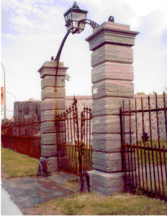
Figure 2.10 Côte-des-Neiges reservoir site entrance gate, 2001
