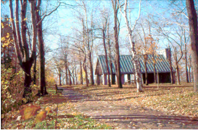
Figure 6.2 Summit reservoir, pumping station and picnic shelter, 2001
