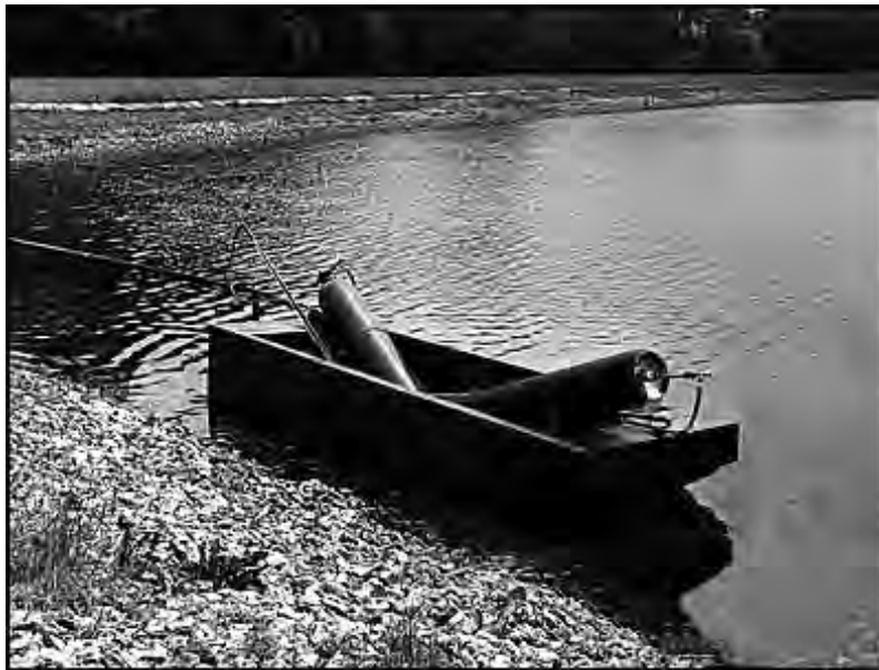
Figure A.25 Chlorine dispensing boat and apparatus, 1955
