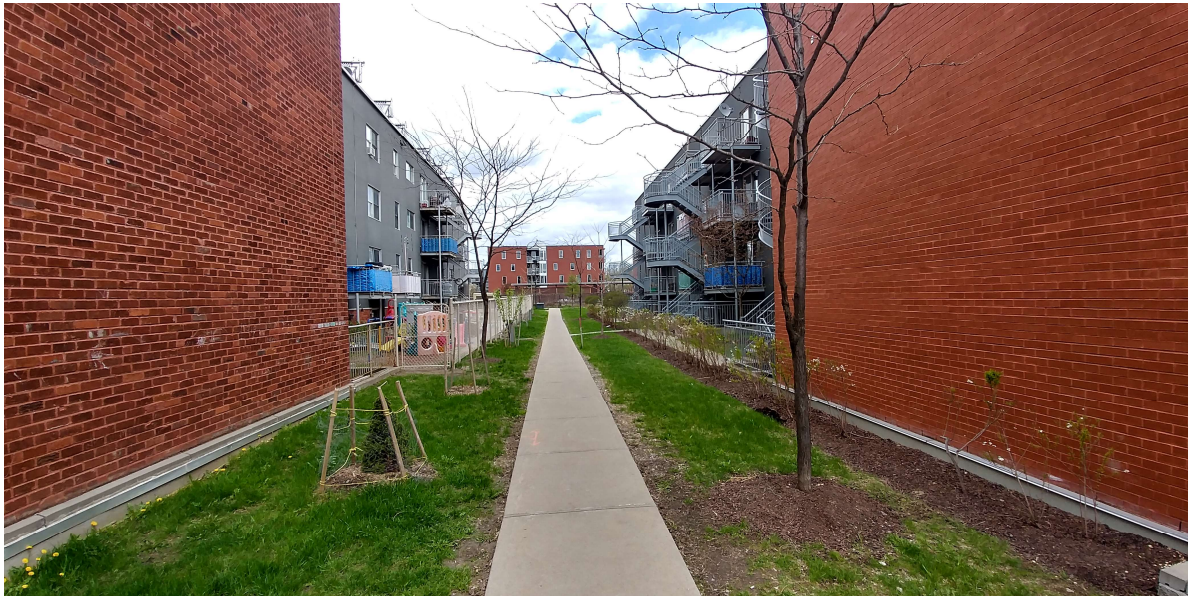
Figure. 5 – The difference between re-used bricks and newly installed bricks.
