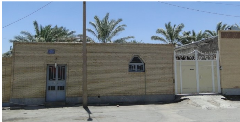
Figure 3.2: An example of the ODR reconstructed houses – Photo by: M. Fayazi
