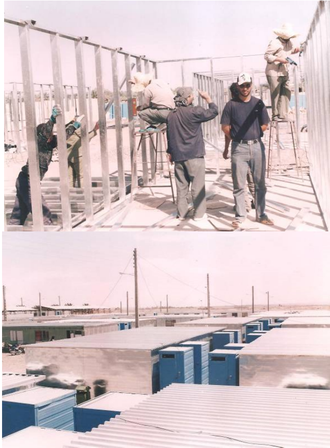
Figure 4.3: Camps consisting of prefabricated units – Photos by: M. Fayazi
