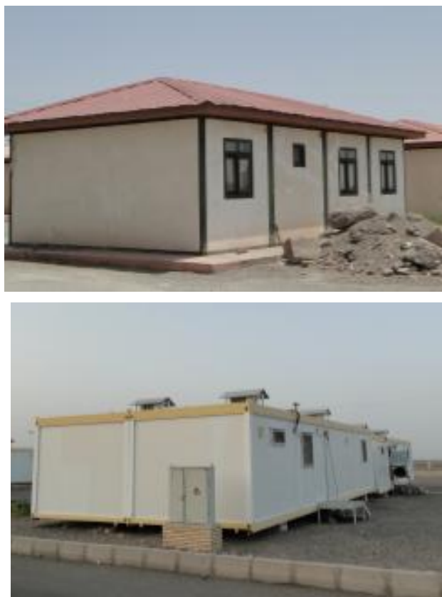
Figure 4.6: Complete high-quality units – Photos by: M. Fayazi
