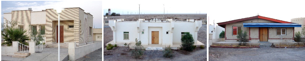
Figure 2.5: Some of the sample houses provided and exposed by different companies and NGOs –
