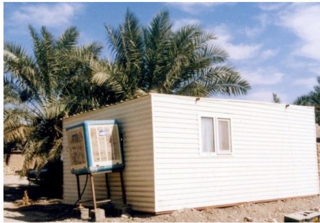
Figure 4.5: Prefabricated units assembled in the yard of destroyed houses – Photo by: M. Fayazi
