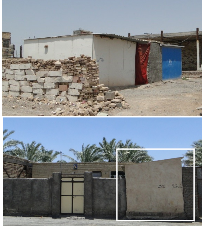
Figure 3.3: Pre-fabricated temporary units (up). Temporary units made of masonry materials (down) – Photos by: M. Fayazi.
