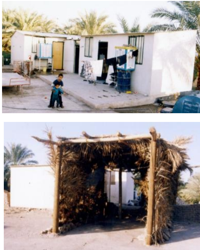
Figure 4.7: Modified temporary units by their inhabitants (up), and expanded temporary units using local materials (down) – Photos by: M. Fayazi
