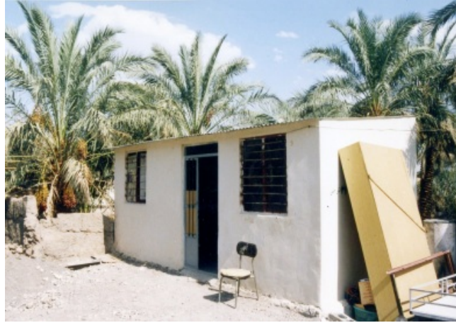
Figure 4.4: Units made of steel frame and masonry walls in the yard of destroyed houses – Photo by: M. Fayazi
