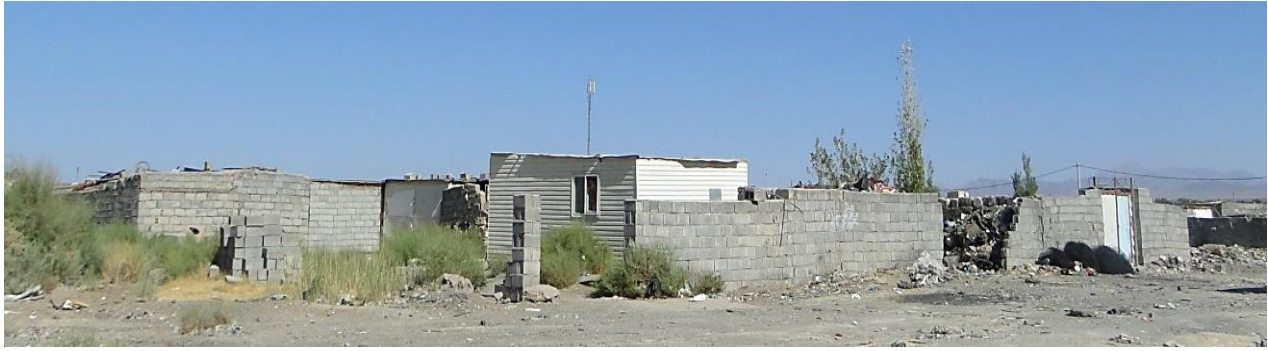
Figure 3.5: Informal settlement (Janbazan) in the outskirts of the city – Photo by: M. Fayazi.
