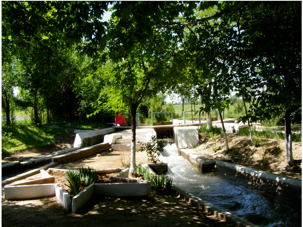
Figure 7 Distribution infrastructure at the head of the system
