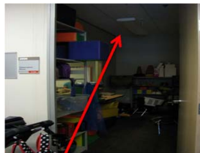
Broken light bulbs in some observation rooms
