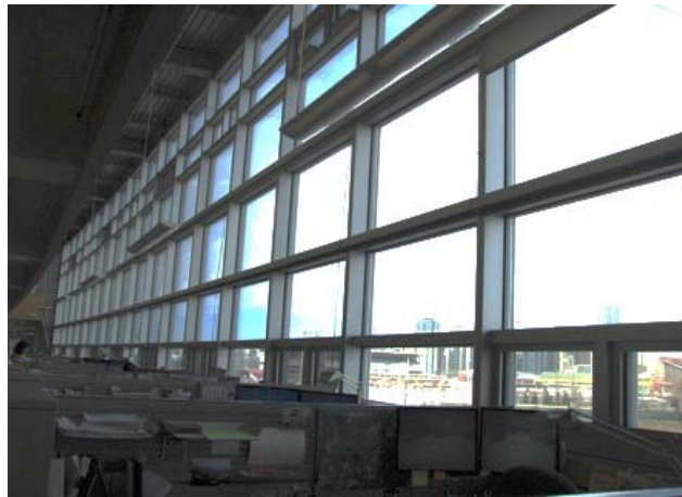
Figure 73. Northern windows into the WCB
