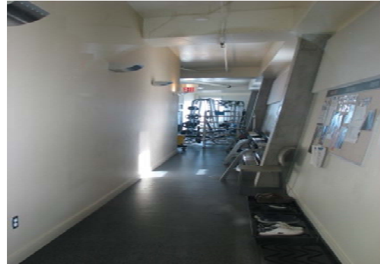
Figure 98. Gym hall in the WCB
