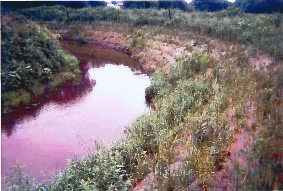
Figure 3: Soft-engineering stabilization technique (using vegetation) implemented in June 2003 in the study reach.
