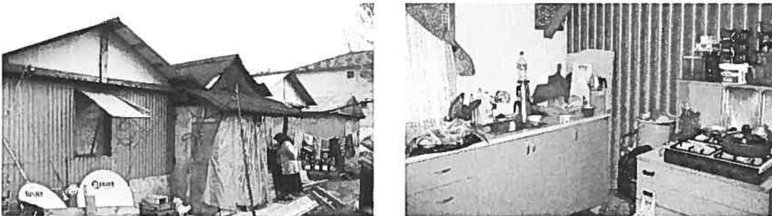
Figure 39 Two paper temporary houses are consolidated into one dwelling with the addition of a kitchen and bathroom in the middle. Outside view of the house (left) and inside view of the kitchen built between to the two paper houses (right).
