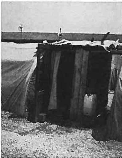
Figure 17 Example of winterised tent additions
