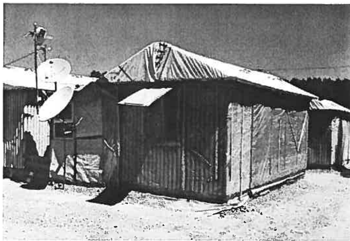
Figure 15 Paper temporary houses in Turkey
