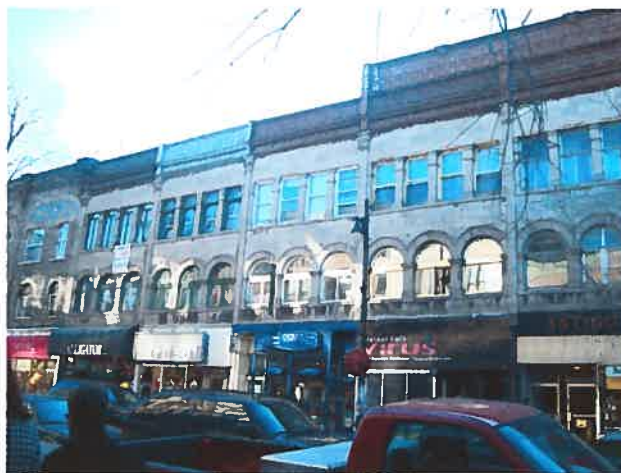
Figure 57 : Le 3640-3712, boulevard Saint-Laurent, le Baxter Block.
