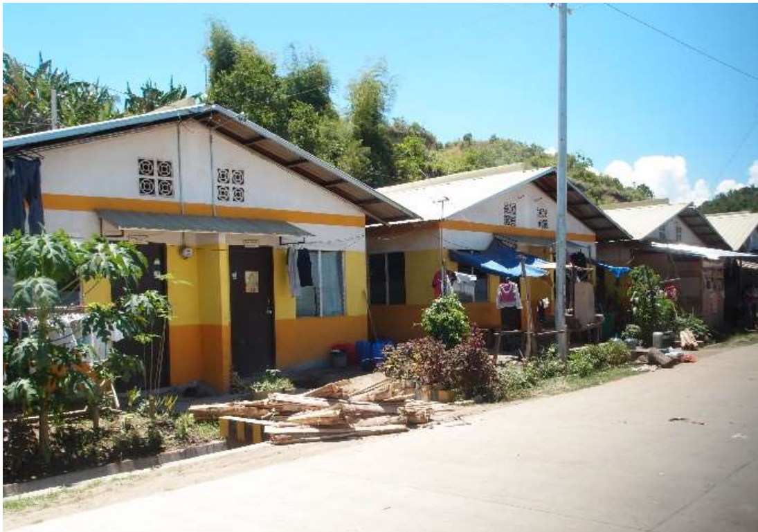
Fig. 6.8. Habitat for Humanity Philippines-built relocation housing just before residents move in (27 November 2012, top) and several weeks after residents have moved in (19 March 2013, bottom).
