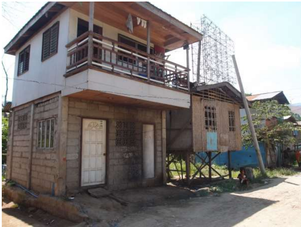
Fig. 6.10. Renovations made to houses affected by Sendong floodwaters. A build-back-taller strategy was adopted by both middle class and urban poor survivors who built an upper floor with a so-called “panic room” (10 March 2013).
