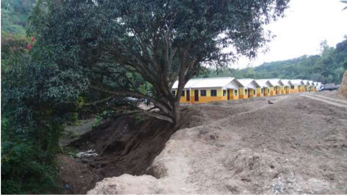
Fig. 6.6. Relocation houses built between a steep landslide-prone hill (on the right) and a live creek (on the left) that floods nearby areas during the rainy season.
