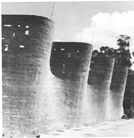
Figure 39 Murs en construction.
