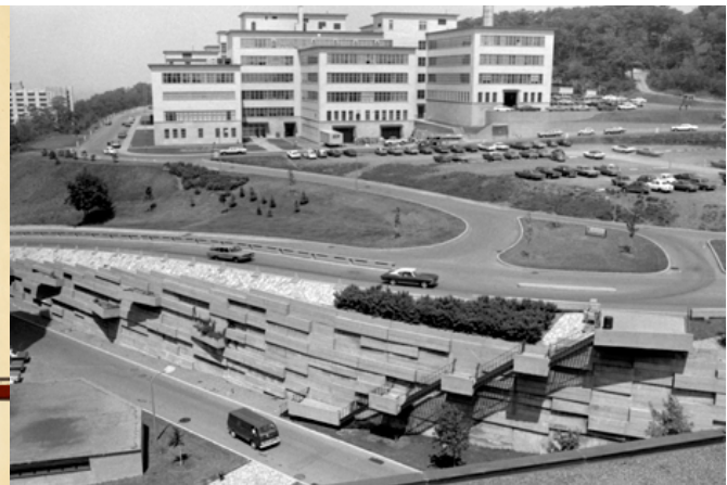
Figure 8 The photo shows the original retaining wall designed by the artist Jean-Noël Poliquin and its relationship to the slope of the mountain and to the roadways. Part of it still exists today. Source: Université de Montréal – Plan d’ensemble [entre 1960 et 1980]. Université du Québec à Montréal. Service des archives et de gestion des documents. Fonds d’archives Jean-Claude-La-Haye, 63P1/734 (27.00)
