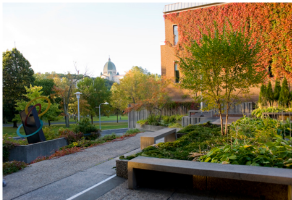
Figure 16 The areas to the south of the Maximilien-Caron pavilion have conserved their authenticity, evident here in the concrete benches, the low walls, and the slabs of exposed aggregate concrete. Photo: Denis Farley, 2010.
