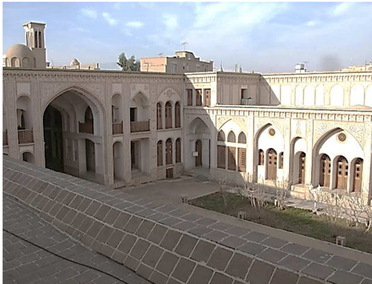
Figure 2-2: The southern face of courtyard, Ameri house, Kashan, Iran. Photo courtesy of author
