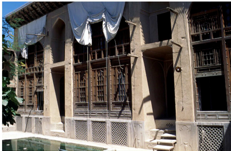
Figure 2-6: The exterior view of three-door room, Yazd, Iran
