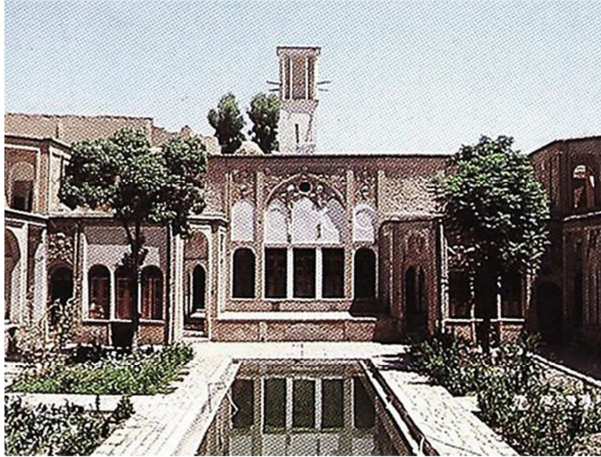
Figure 2-23: Pool and plants in front of northern side. Photo courtesy of cultural heritage organization of Iran
