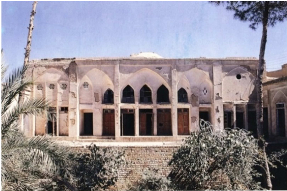
Figure 3-14: The northern side of courtyard, case no. 1 (Al-e Yasin house), Kashan, Iran. Retrieved from Haji-Qassem (1996)
