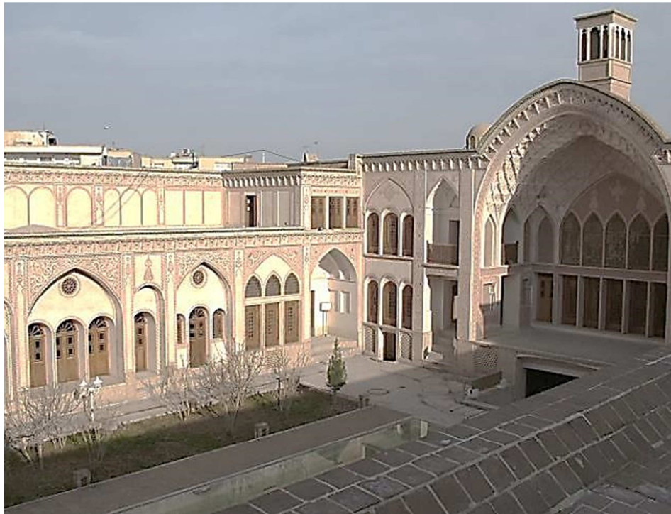
Figure 2-3: The northern face of courtyard, Ameri house, Kashan, Iran. Photo courtesy of author
