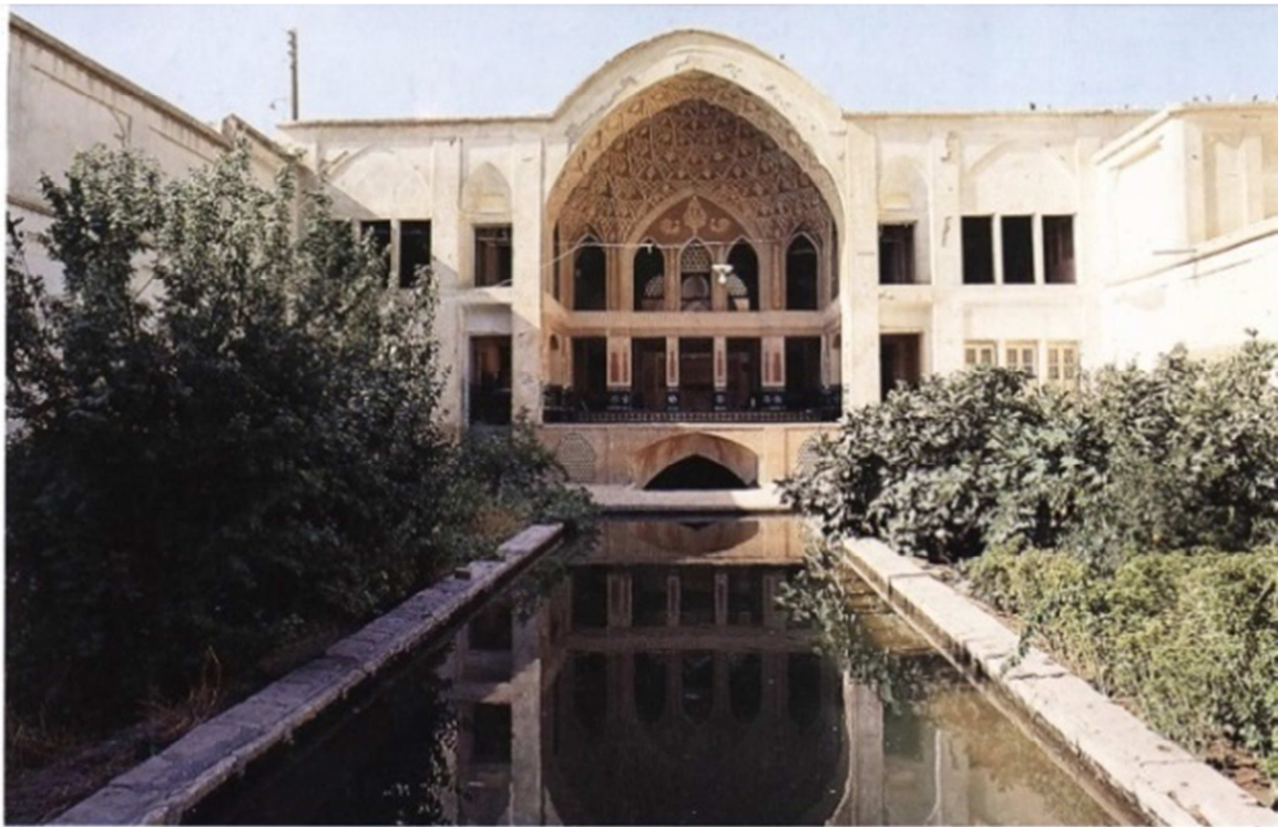
Figure 3-20: The southern side of courtyard, case No. 3 (Sharifian house), Kashan, Iran. Retrieved from Haji-Qassemi (1996) and edited by author.
