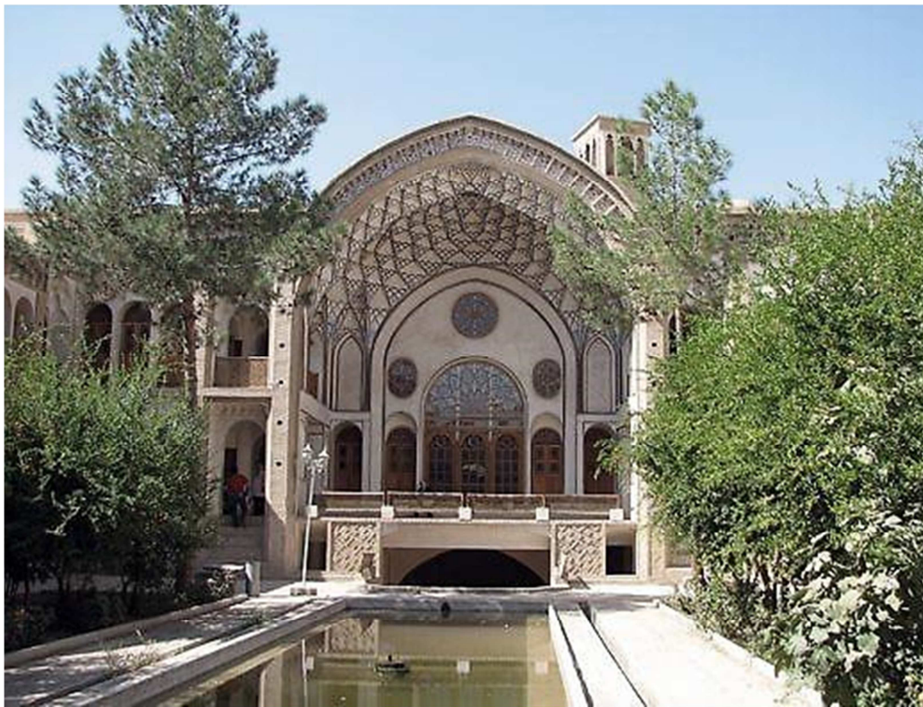
Figure 2-22: Pool and plants in front of northern side, Ameri house, Kashan, Iran. Photo courtesy of cultural heritage organization of Iran
