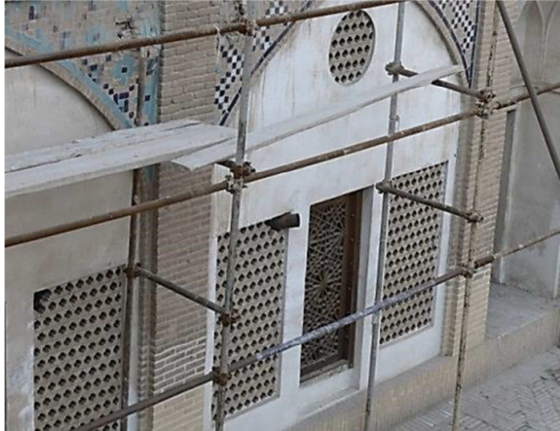
Figure 2-17: Wooden and brick lattice openings for preventing the penetration of direct sunlight into spaces. Photo courtesy of author
