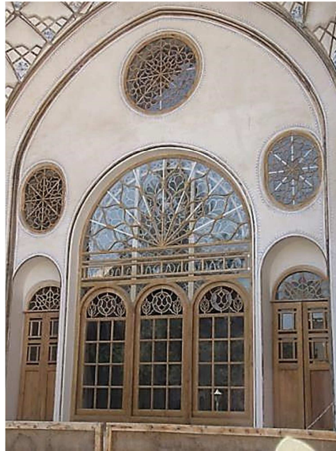
Figure 2-15: The exterior view of lattice and coloured openings, Ameri house, Kashan, Iran. Photo courtesy of the cultural heritage organization of Iran
