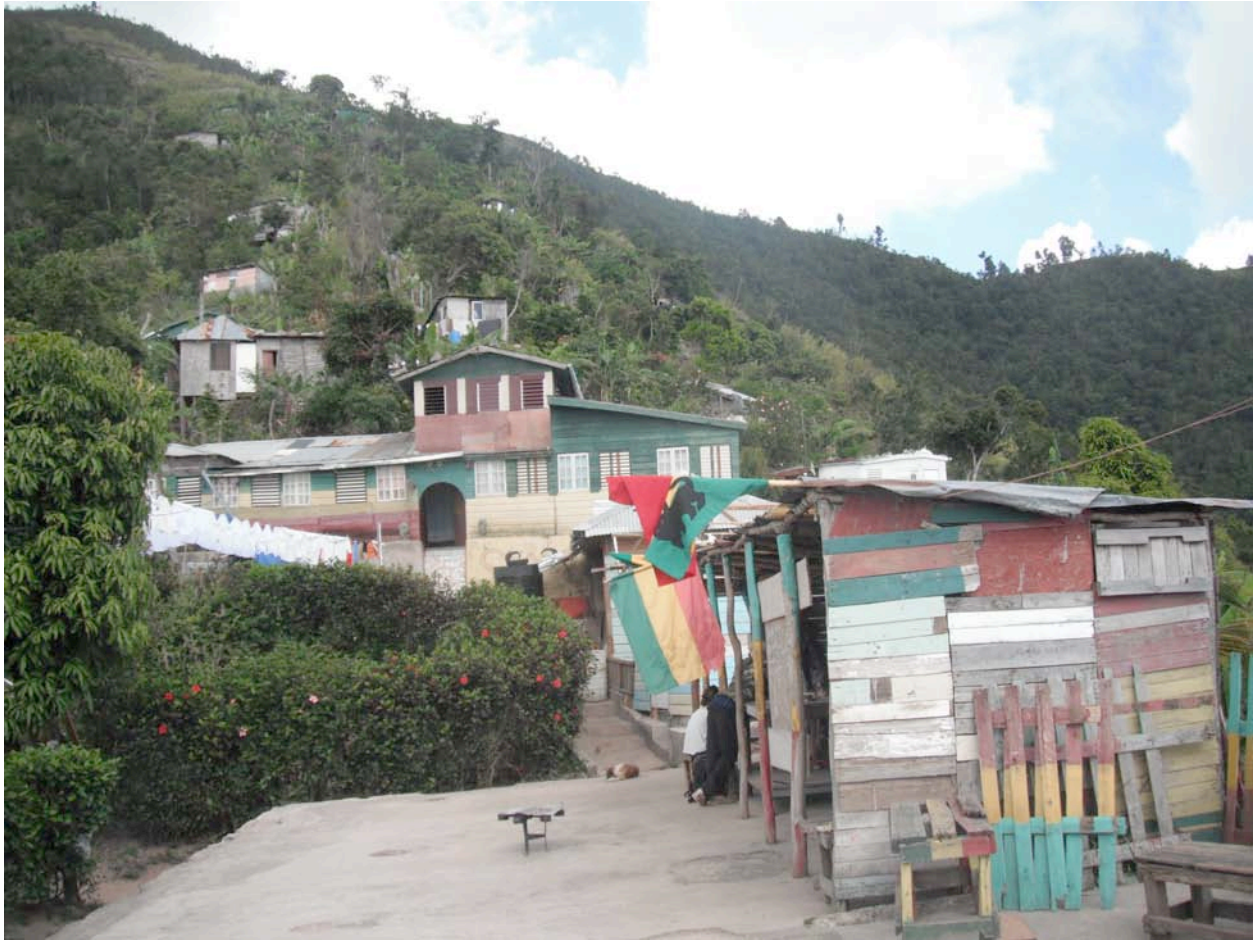
Figure 45: Residences (back) and School (front) at Mount Zion Hill Temple (Blue Mountains, Saint Andrew Parish, Jamaica, April 22, 2011)
