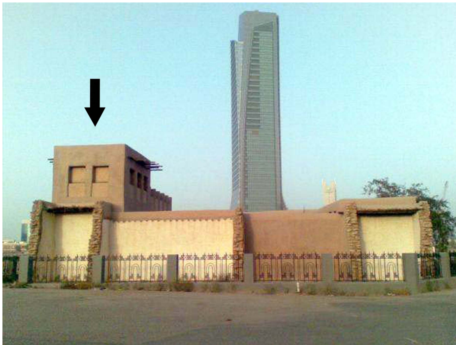
Figure 8: Badgir of one of the heritage buildings in Kuwait City. The Al-Babtain Waqf Culture Tower is in the background (source: researcher, 2011-01-18).
