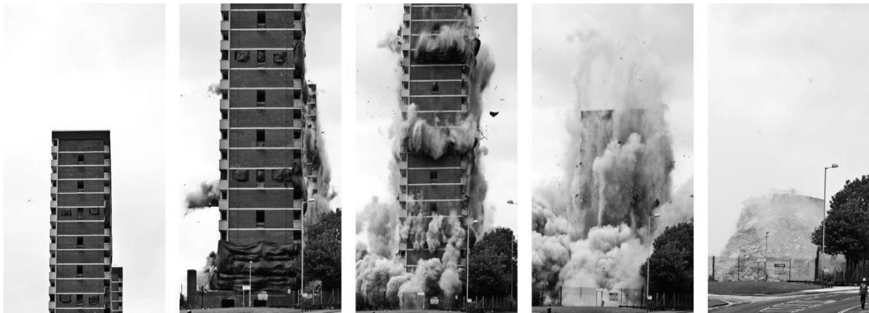
Figure 1.6. Sequence of demolition
