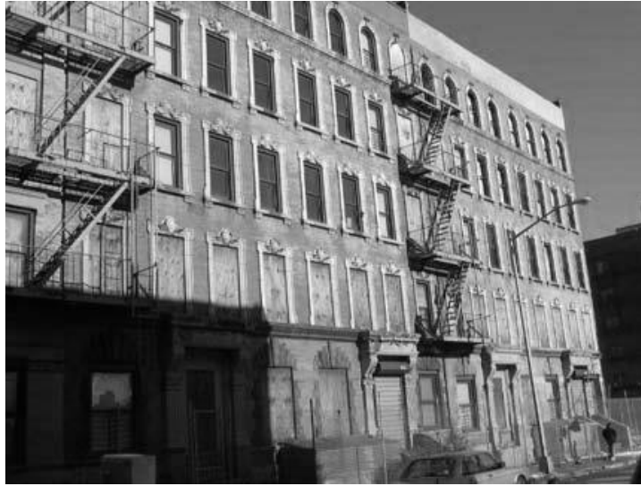
Figure 1.8. Obsolete apartments (Laughlin & Johnson, 2011)
