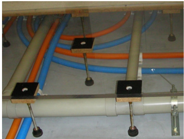
Figure 6.30. Kodan SUPPORT & INFILL (KSI), raised floor components, Tokyo, Japan
