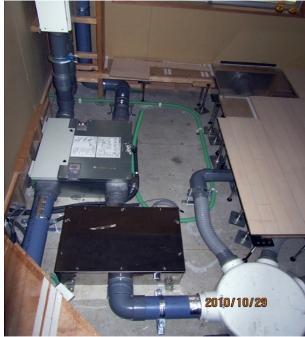
Figure 6.29. Kikou SUPPORT & INFILL (KSI), raised floor
