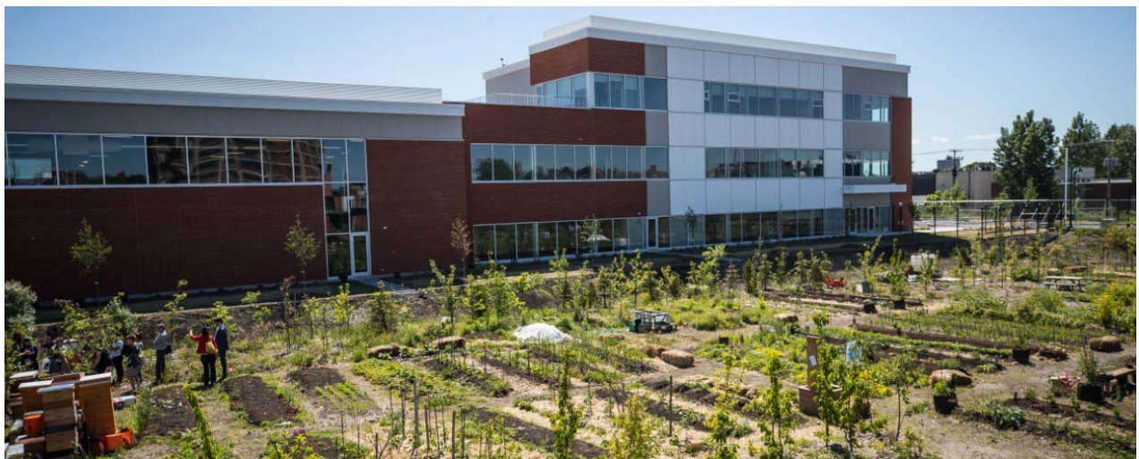
FIGURE 25 COUR DE SERVICES OUTREMONT
