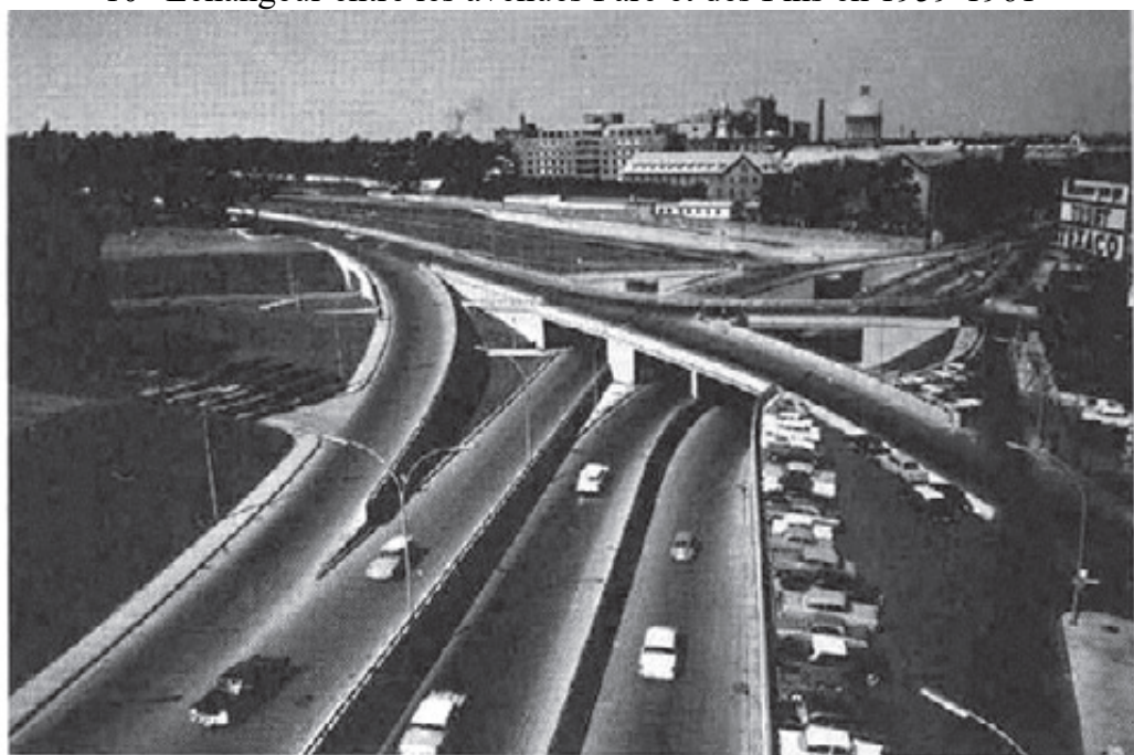
Pine-Park Square: grade separation between Pine and Park Avenues – Park Avenue shown in the left background carries more than 40,000 vehicles per day.
