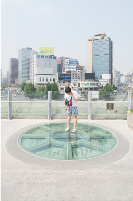
Figure 59. View of windows revealing the visible signs of age in Seoul's reinforced concrete structure. Created by Ossip van Duivenbode, 7 October 2019. https://www.archdaily.com/882382/seoul-skygarden-mvrdv .
