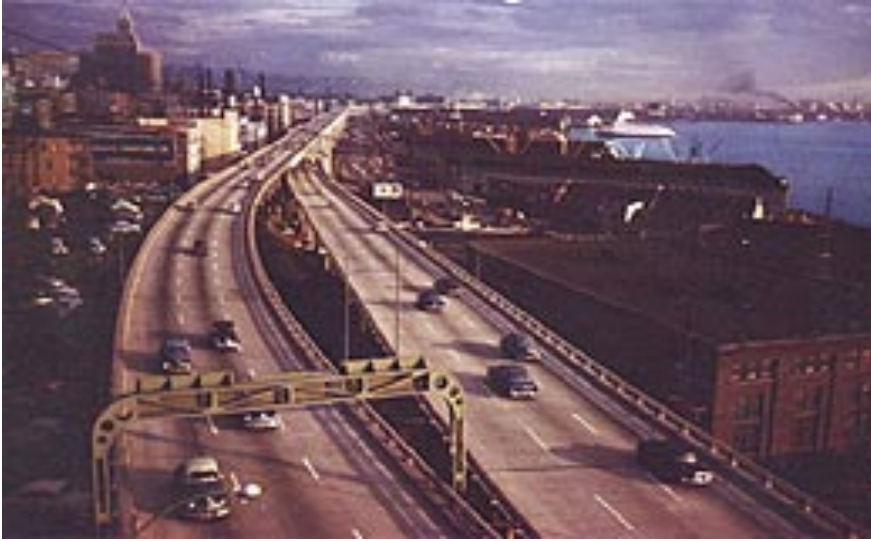
Figure 63. Postcard view of newly completed Alaskan Way Viaduct in the 1950s. From History Link online Encyclopedia of Washington State History, courtesy of Seattle Municipal Archives. http://historylink.org/File/9982
