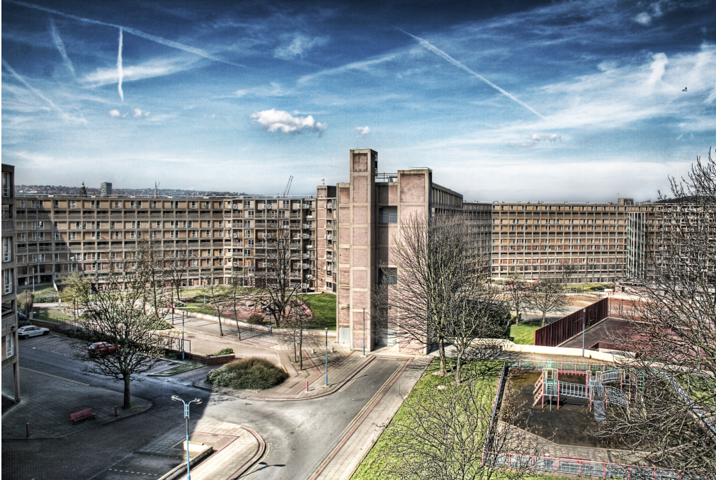
Figure 21. Park Hill Estate, 1961, Sheffield, UK. Photo by Henk Snoek. Photo by Paolo Margari, 2007. From Wikimedia Commons. https://commons.wikimedia.org/wiki/File:Park_Hill,_half-abandoned_council_housing_estate,_Sheffield,_England.jpg
