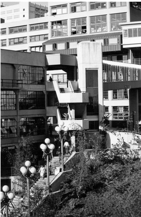
Figure 64. "Hill Climb" constructed in 1977 to link the waterfront to Pike Place Market. From History Link online Encyclopedia of Washington State History, courtesy of Seattle Municipal Archives. http://historylink.org/File/10666
