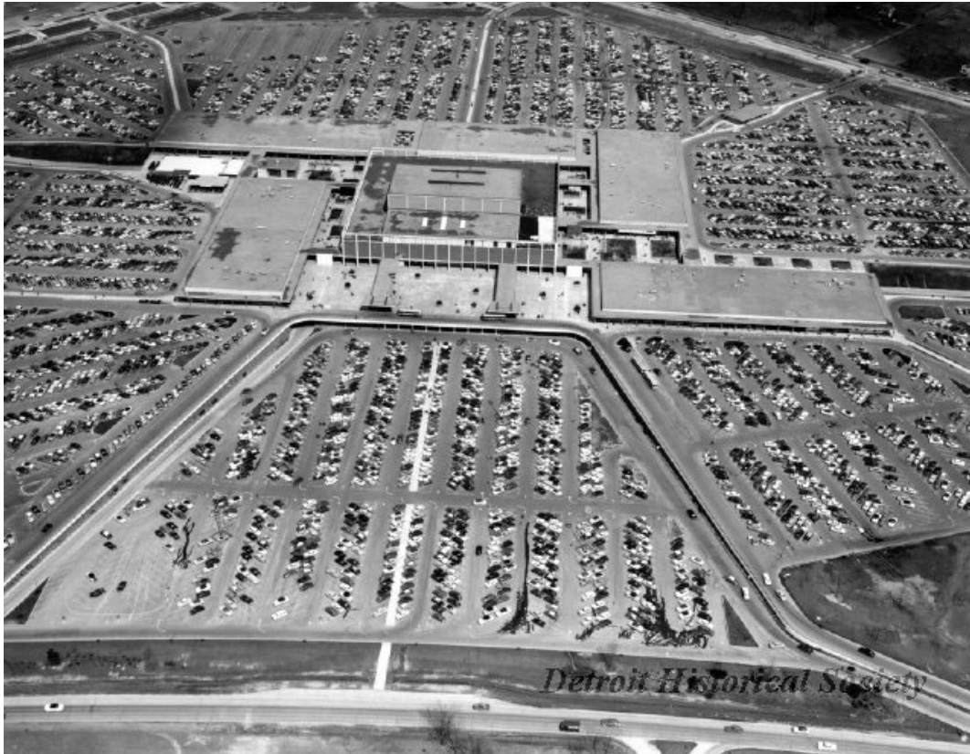
Figure 19. Northland Shopping Center, Gruen Associates, 1952-54, Southfield, Michigan. Photo by York Photographic Studios, 1954. From Detroit Historical Society. https://detroithistorical.pastperfectonline.com/photo/C53D0960-95DF-43E0-9C1E-422989956384
