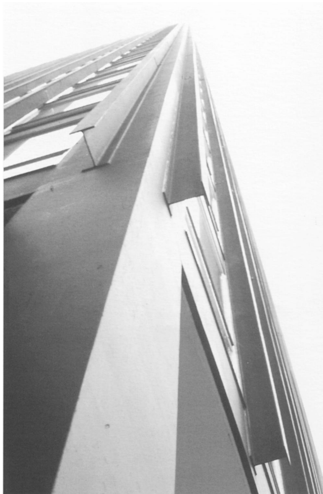
9. Ludwig Mies van der Rohe, Lake Shore Drive Apartments, Chicago, Illinois, 1949–51, view of corner I-beam.
