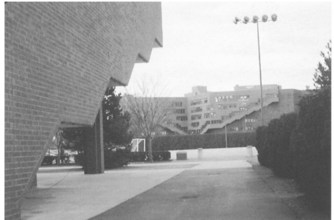
4. Davis and Brody, MIT Hockey Rink and Field House, Cambridge, Massachusetts, 1980–81, view of corner reflecting, in the background, Aalto's Baker House Dormitory, 1947–49
