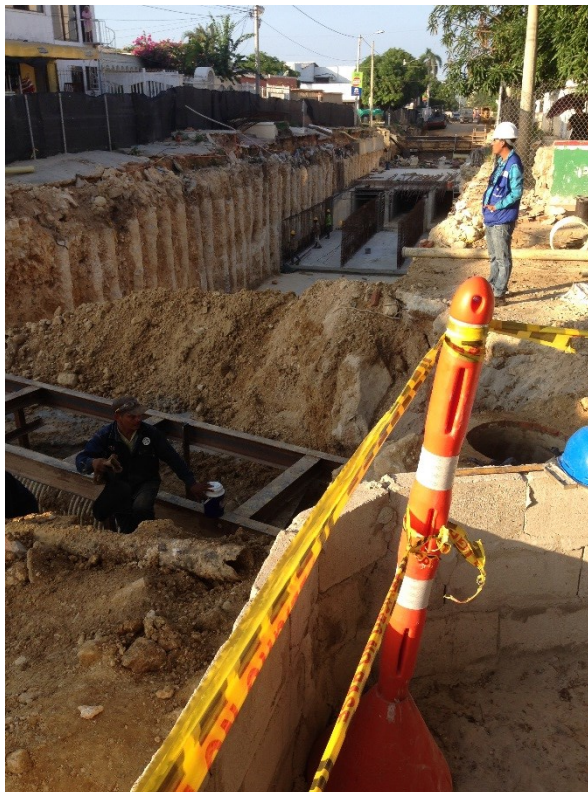
Figure 12 – Storm drain. Detail.
