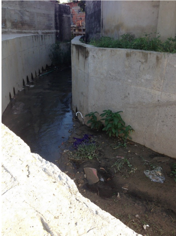
Figure 11 – Storm drain. Detail.
