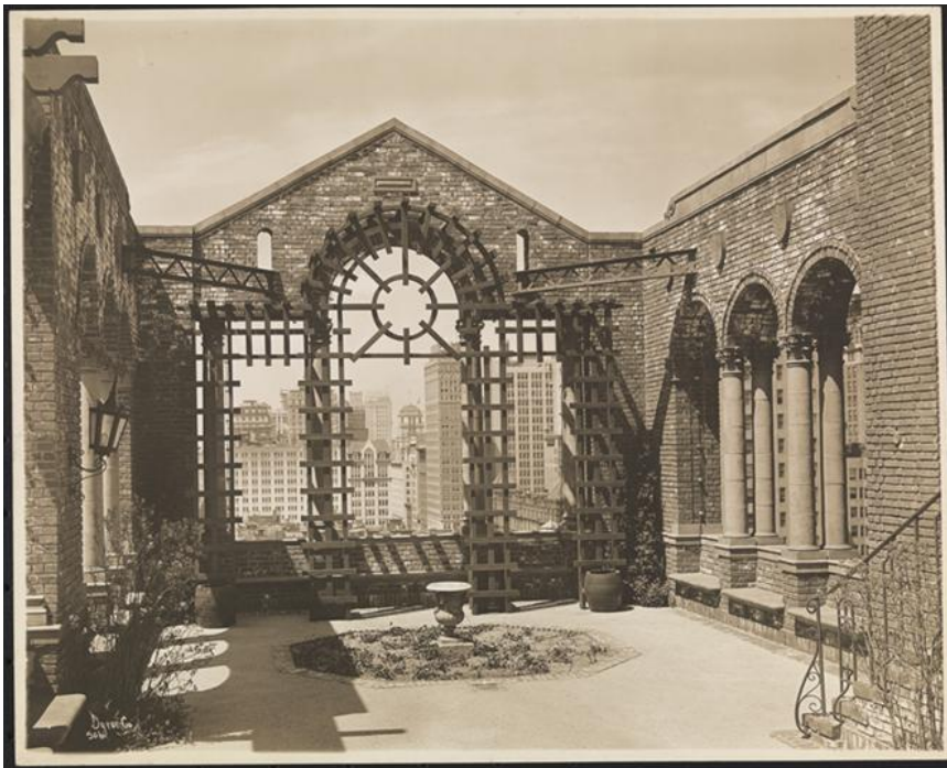
Figure 193 - Le roof garden de la Allerton House, 1919
